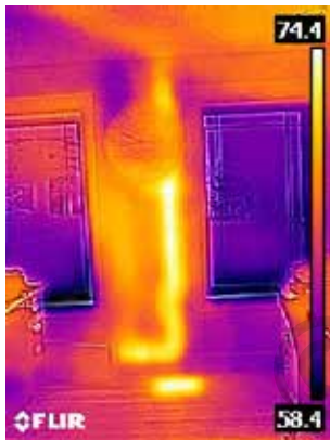
Warm drain pipe in wall
